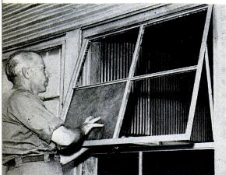
Alpyrite Company of America photos Above, flat-type translucent plastic may be used in place of regular frosted glass where vision is not desired. Below, panels of corrugated plastic, 10 or 12 ft. long, simplify construction of a carport roof
